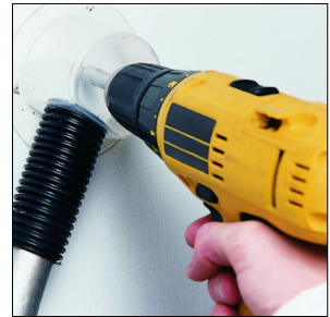
Control measures: shadow vacuuming and using plastic enclosures as local extraction
