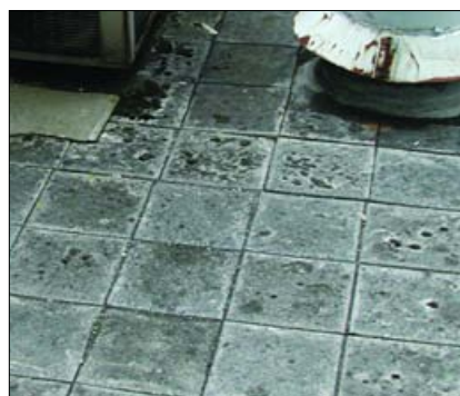
Asbestos cement tiles on a roof
