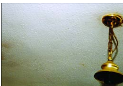
Textured coating on a ceiling
